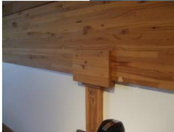
2h Fire Rated Connection The Landing, Vancouver
