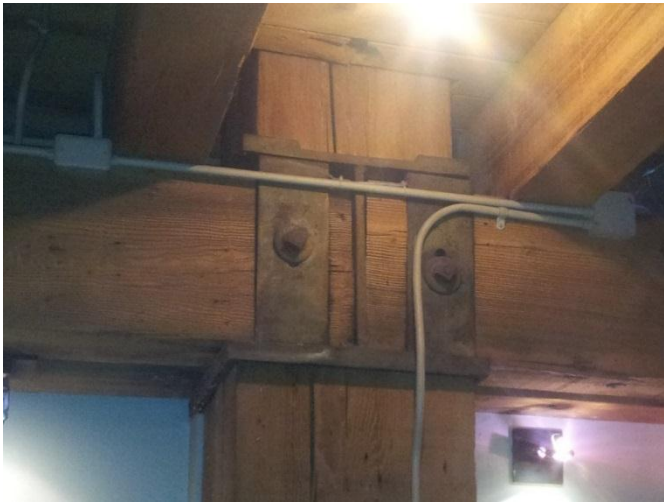
2h Fire Rated Connection The Landing, Vancouver
